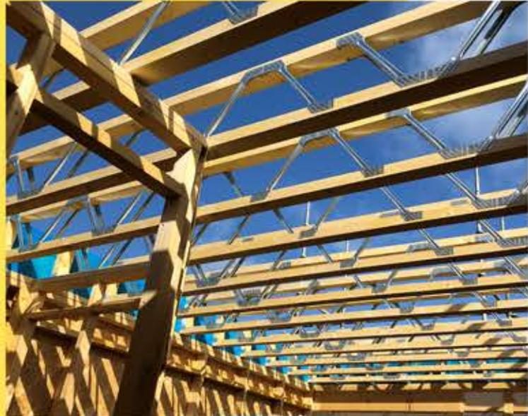
The Posi-Joist allows a variety of internal room layouts within an external shell due to its clear spanning capabilities. The Posi-Joist does not just joist floors; it can adequately span for flat and pitched roofs. Its span capability and timber flanges make it the more desirable alternative to all steel systems. The unique open web design makes installation of services and utilities far simpler and quicker resulting in a reduction in both labour costs and build time on site.
